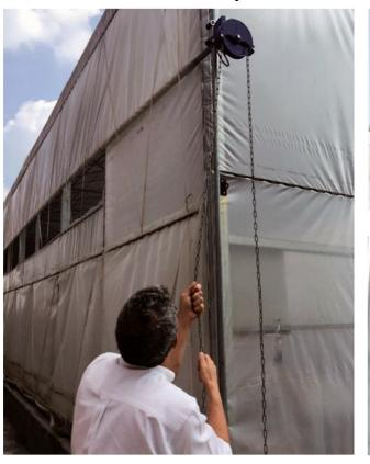
HIGH SIDEWALL ventilation of Poly Greenhouse
