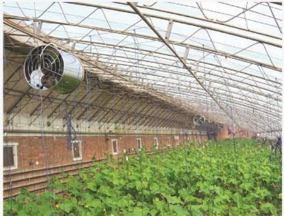
Since the Greenhouse is a relative close environment , the air in the greenhouse is not easy to flow , and the temperature and humidity in the greenhouse air normally high. It can easily breed warious pests and diseases in such an environment. In order to improve the environment inside and keep the air in the greenhouse flowing, Beijing Fenglong meticulously designed and producted the FLC<sup>®</sup> circulation fan.
